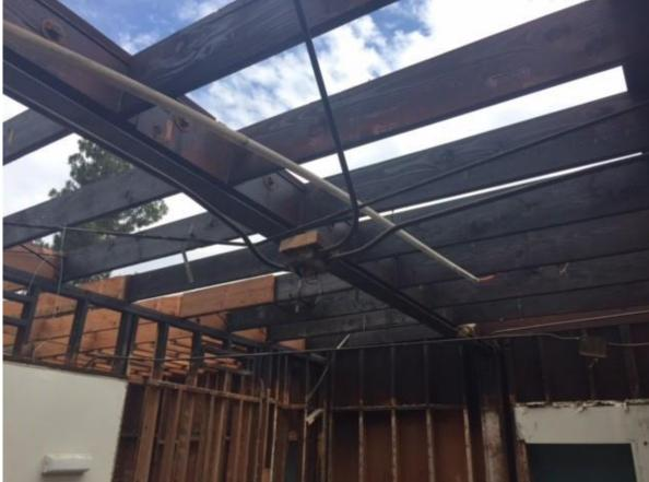
Old fire damage discovered during construction
