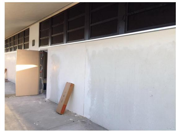
New concrete placed, stucco to match existing building exterior, New windows and frames
