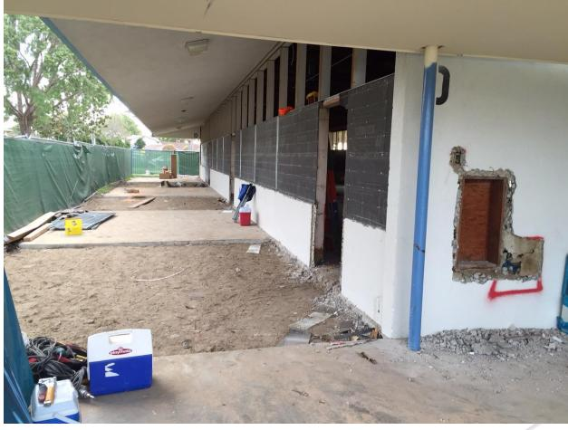
Old non- compliant concrete removed, windows infilled for safety
